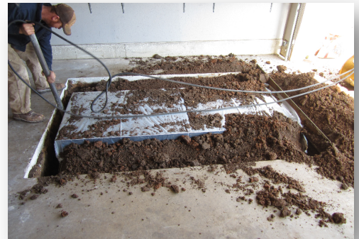
Hydraulic tamping – it's just one of the extra steps we take to ensure a lifetime product. Many competitors simply set the surrounding dirt in by foot.
