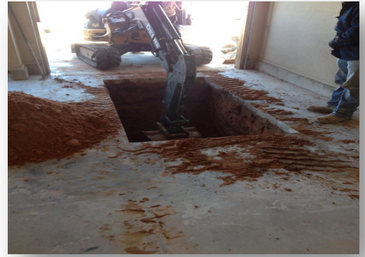
Installer digs hole for shelter placement. Typically installed 1 foot from garage
