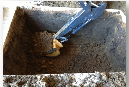
Work site is kept clean before, during and after installation.
