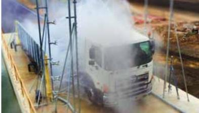
One of the most popular engineered solutions is a combined LV / HV wash system with a manual HV wash pad for larger vehicles.
