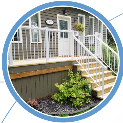
FRONT STAIR AND LANDING
