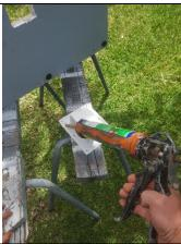
Step 9: Install the CAVGUARD plumb in the wall opening using an appropriate sealant/adhsieve to seal and adhere the CAVGUARD to the wall face of the lining.
