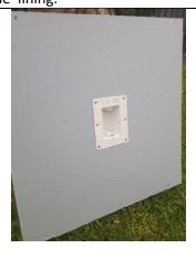
Step 11: Seal any cable entries into the CAVGUARD and Waterproofing the wall linings and the CAVGUARD to form a continuous membrane in accordance with the manufacturers instructons. Ensure that the
