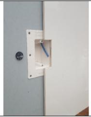
Step 12:Install wall finishes in accordance with the manufacturer's instructions, cutting an opening of a size so that access to the threaded inserts is maintained and the wall outlet wholly covers the opening once installed
