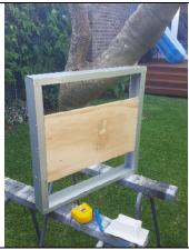
Step 1: Install a plywood noggin, minimum 12mm thick and 300mm in width. Centre the noggin vertically with the intended location of the CAVGUARD and flush with the face of the wall framing
