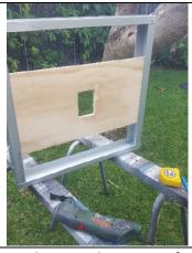
Step 4: Using the centrelines as a reference, cut a clear opening 106mm high and 72mm wide in the plywood noggin.
