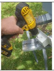
Step 7: If a cable or cables are required to be located within the CAVGUARD, drill a hole within the cable insert zone of the CAVGUARD to suit the cable size.
