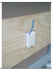
Step 8: Feed the cable of cables form the wall cavity into the hole drilled in the CAVGUARD and place the within the wall opening.
