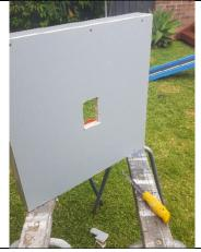
Step 6:Cut an opening in the wall lining to match the opening in the plywood noggin.
