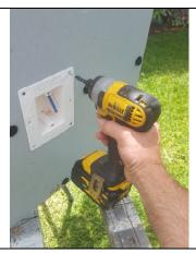
Step 10: Fix the CAVGUARD plumb in the wall opening with x8 off 7g SS countersunk screws, that are of a suitable length to hold securely in the plywood noggin.
