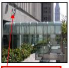
Installed for fall arrest is a selfretracting lanyard attached to a custom anchor above the canopy
