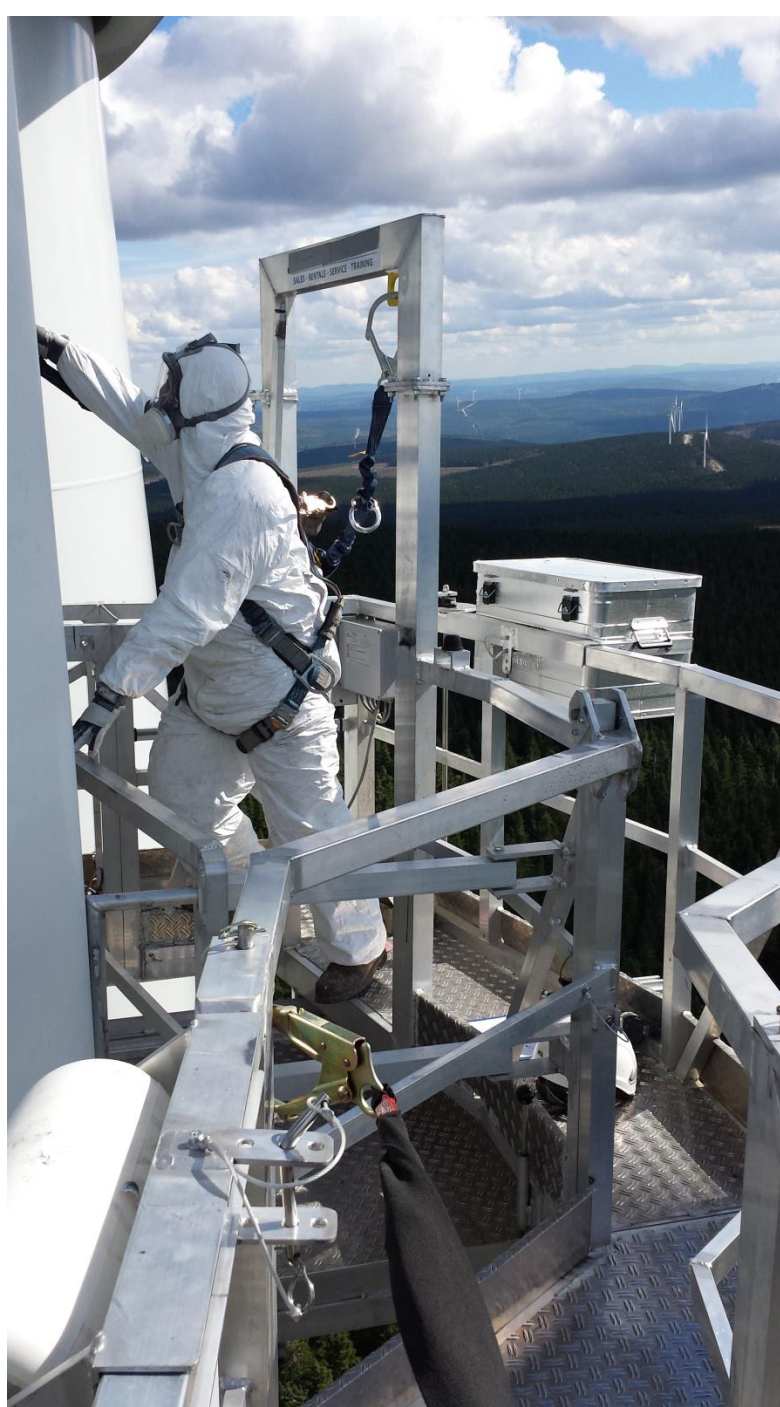
Composite repair from 360 suspended platform
