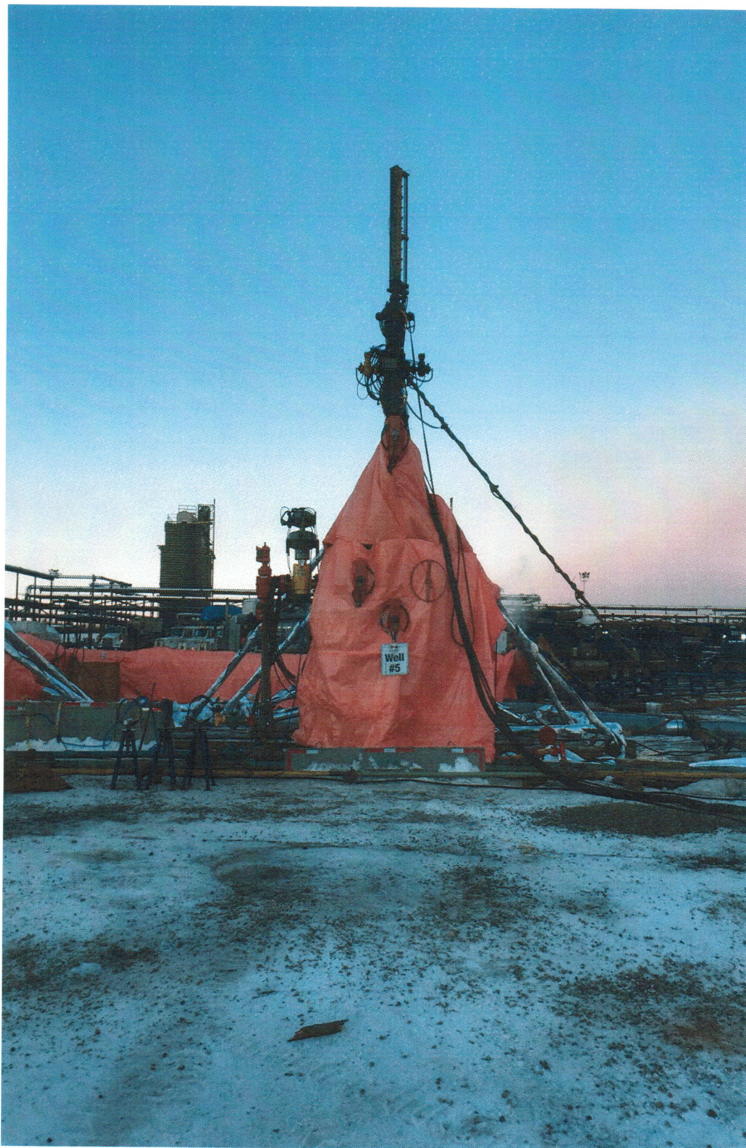
Ball line wrapped with Steam back to fluid pumper, to eliminate cold methanol leaks when displacing frac balls.
