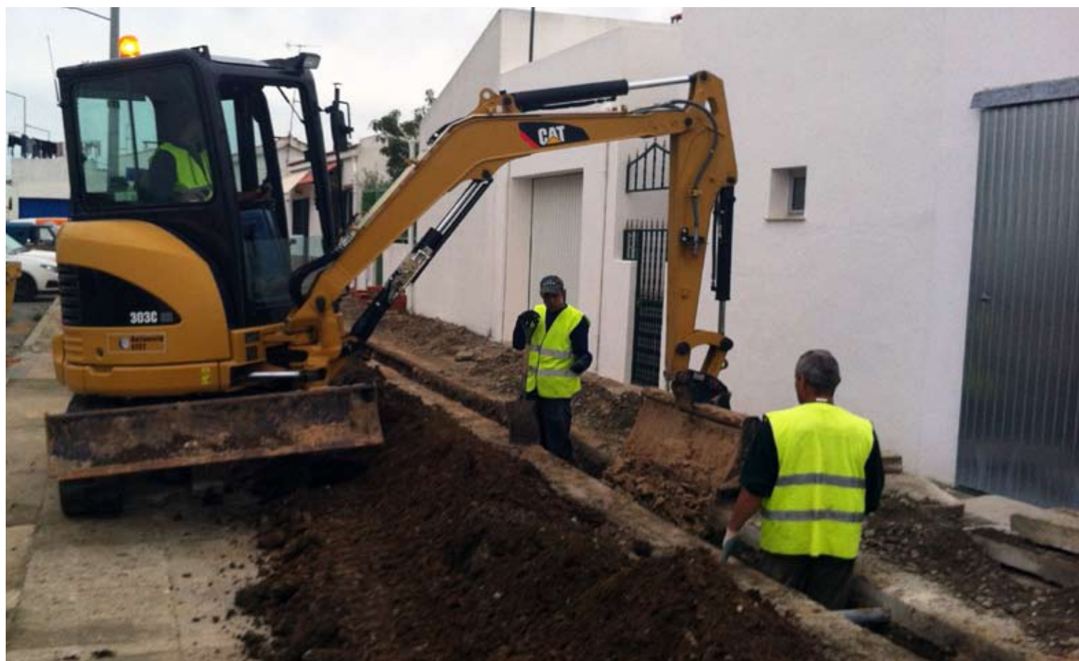
CONSTRUCTION OF POLYETHYLENE (PE) GAS NETWORKS. LISBON (PORTUGAL)
